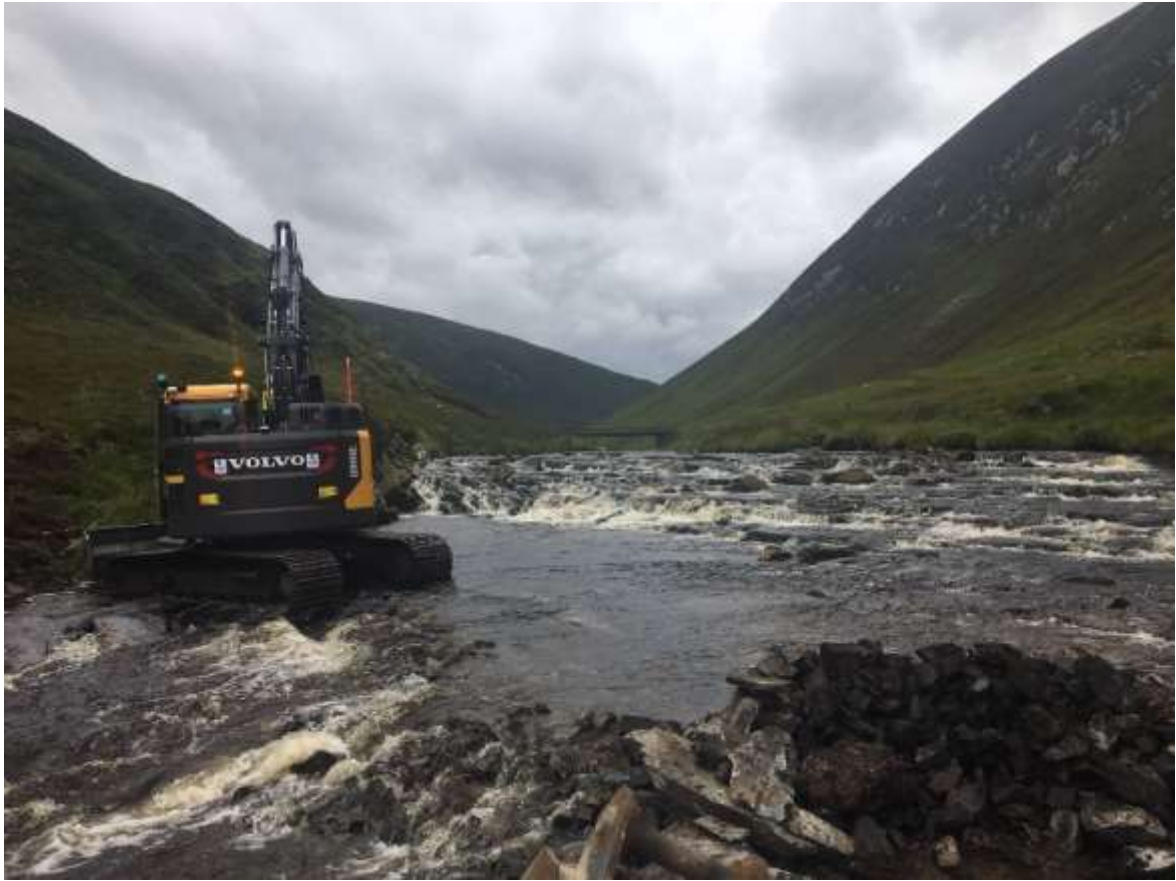
Figure 24 Final remnants of the weir at Deanich being removed.
