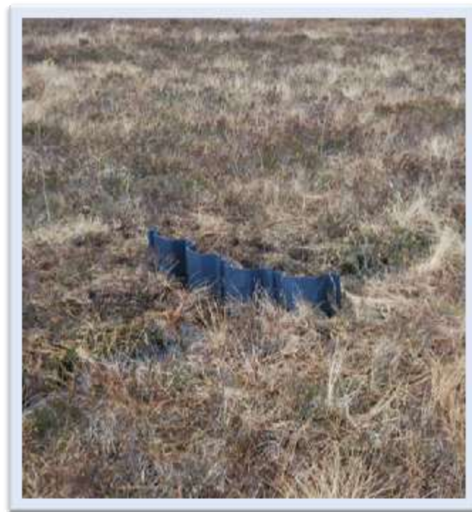
Plastic sheeting used to block drainage ditch.
