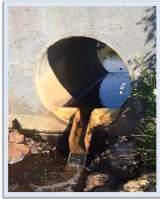
Chute retrofitted onto pipe bridge.
