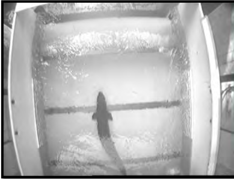
Figure 5.2.7 Adult salmon passing through the counting flume at Shin Diversion Dam (photograph courtesy of SSE)
